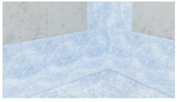
The sealing membrane can be overlapped by 5 cm using the sealing adhesive in the overlap area. Otherwise, the joints can be covered with sealing tape and sealing material. Mix the sealing adhesive and apply it to the waterproofing membrane with a suitable notched trowel. At this point, you can start tiling without further delay.
