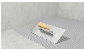
Apply the sealing membrane to the floor precisely and edge to edge, smoothing it towards the edges. Avoid air pockets and glue residue.
